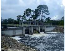
As the water continues down the M-Canal, it passes through Control Structure 4, which can have the gates open or closed depending on the water lev-
